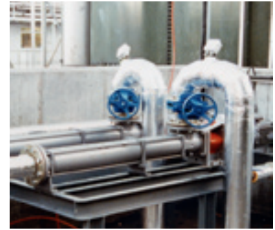
Pumping of slurry mix
