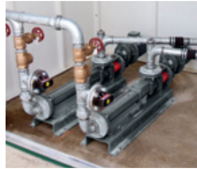
Waste water pumping
