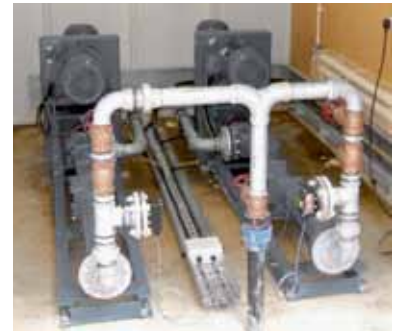
Transfer of raw sewage from a domestic installation
